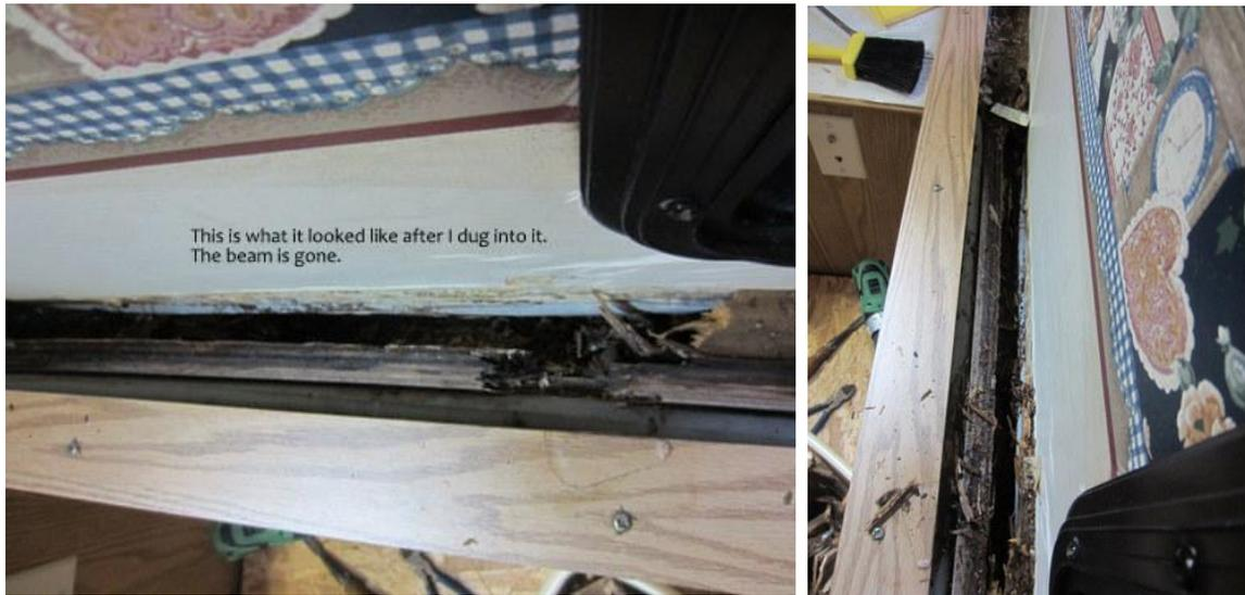
Not only is the beam shown above rotted, but the entire wall below the window was also rotted behind the vinyl wall covering.
