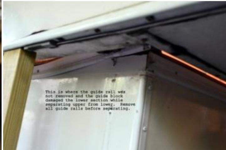
This is where the guide rail was not removed and the guide block damaged the lower section while separating upper from lower. Remove all guide rails before separating.
