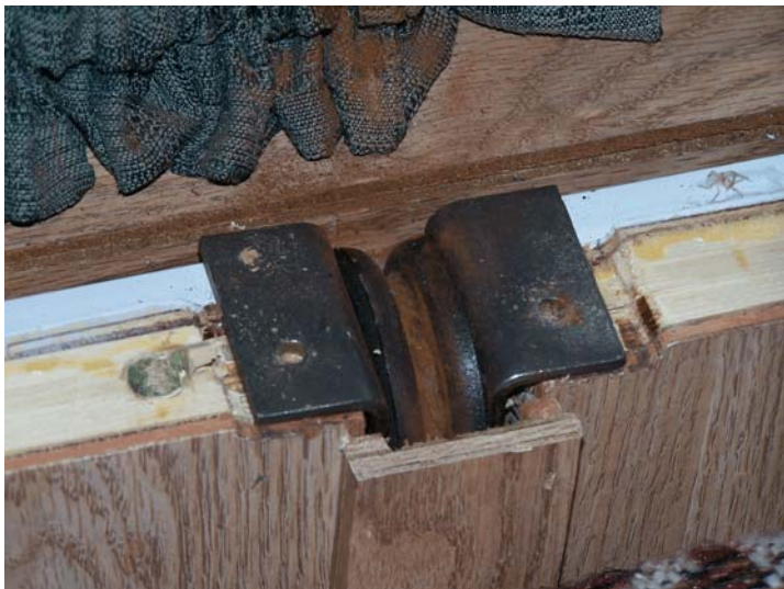
Note the rust where the cable sits on the upper pulley
