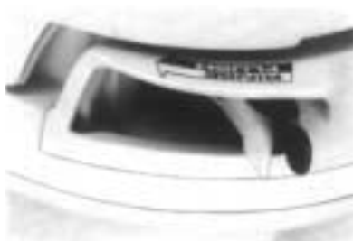
Flushing lever (black) and water fill lever (white) shown in the normal closed position. (Fig. 4-20)
