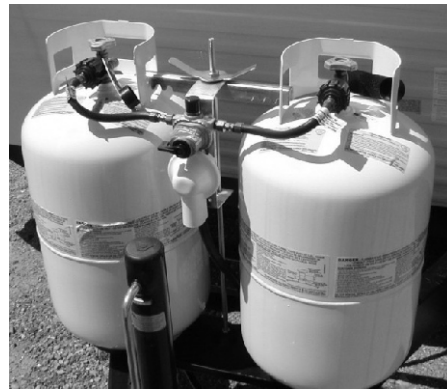
Fig. 4.10 Double cylinder assembly
