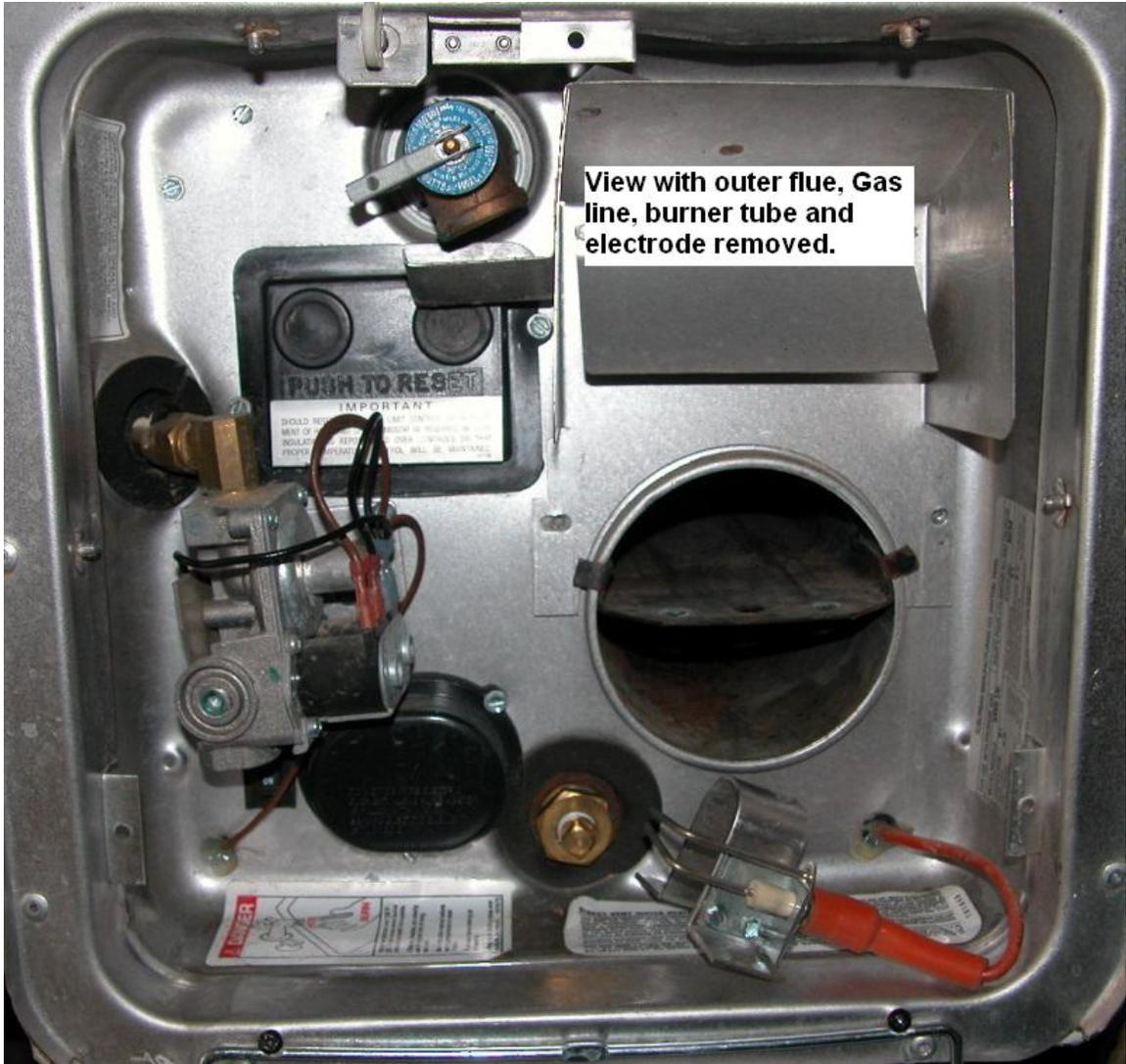
View with outer flue, Gas line, burner tube and electrode removed.
