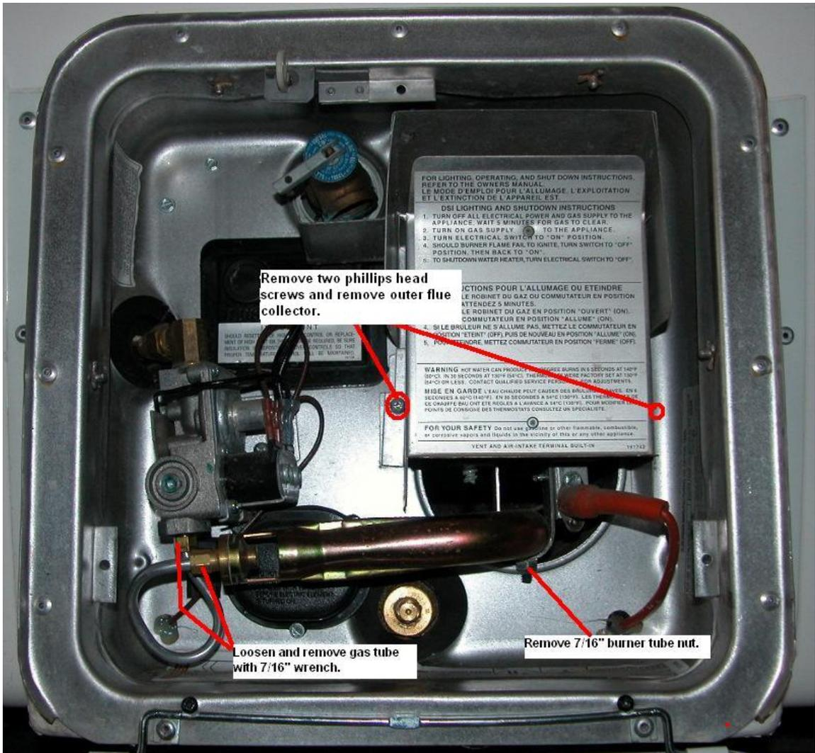
Remove two phillips head screws and remove outer flue collector.
